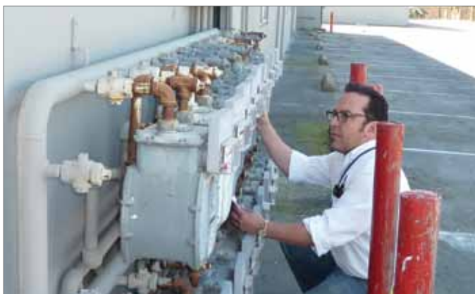
Tommy Young of E3Norcal reads gas meters at Ranch Terrace apartments, a 105-unit complex in Rancho Cordova, a suburb of Sacramento.
